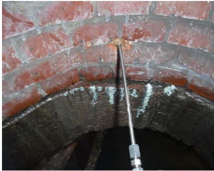
Structure grout injection prior to relining
