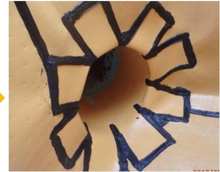
Transition strip from lined pipe to inlet
