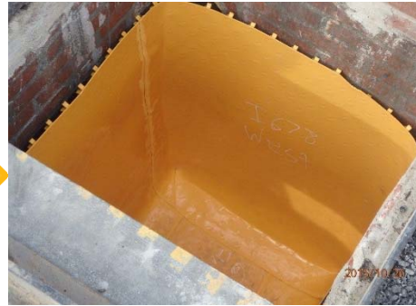
Inlet relining in progress
